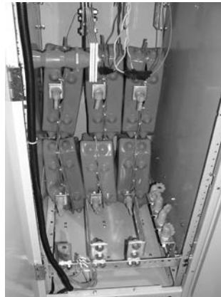
Grounding Balls and Covers
