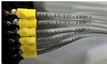
Control Wire Marking
