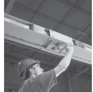
Typical Busway Installation (Torque Indicating Bolt)
